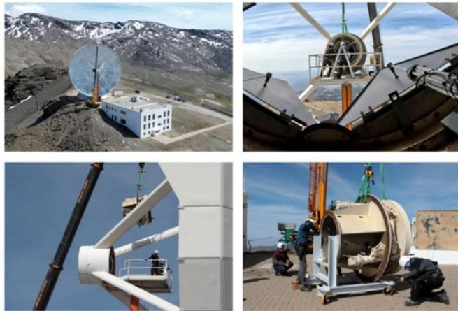
Figure 2: Hexapod disassembly procedures during the servo System upgrade.
